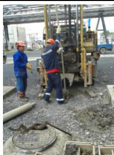
Application-monitoring probe construction
