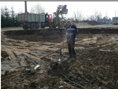
Sample collection during excavation
