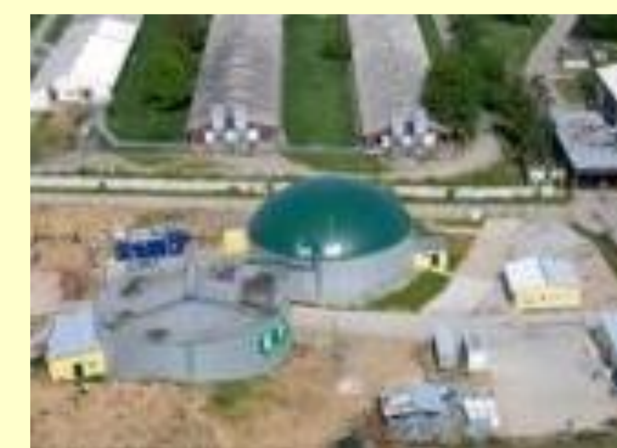
Biogas plant EPS-Nový Dvůr, Kunovice; installation of desulphurization facility,
